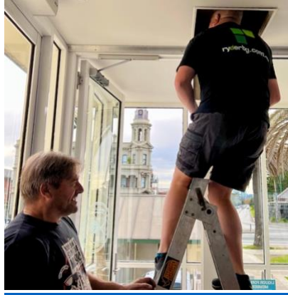
Darren Ryder and Alex Spyrou windproofed the front door.
